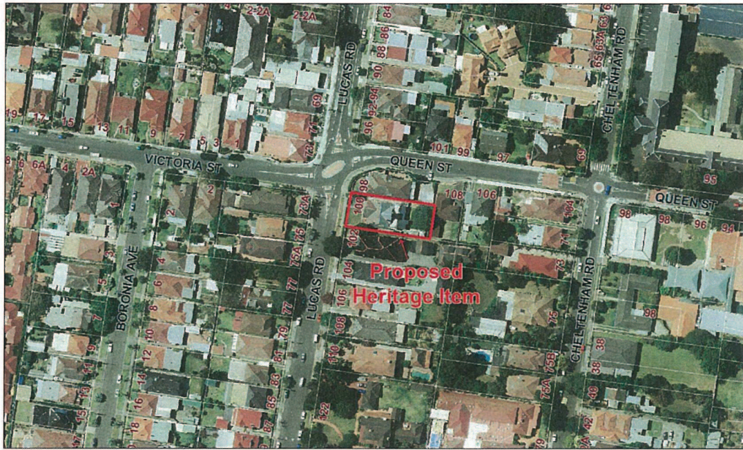
Aerial Photograph of No. 100 Lucas Road Burwood Subject site is shown outlined in red.
